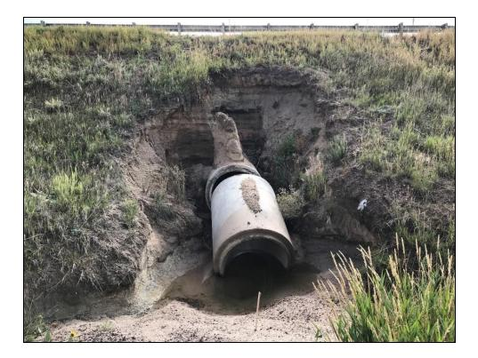
Photo 11.1 Culvert outlet failure on I 25 near milepoint 162.1, 9/6/2018
